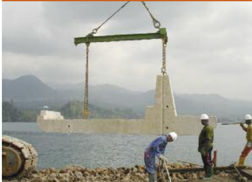
Placing prefab concrete units for maintenance road
