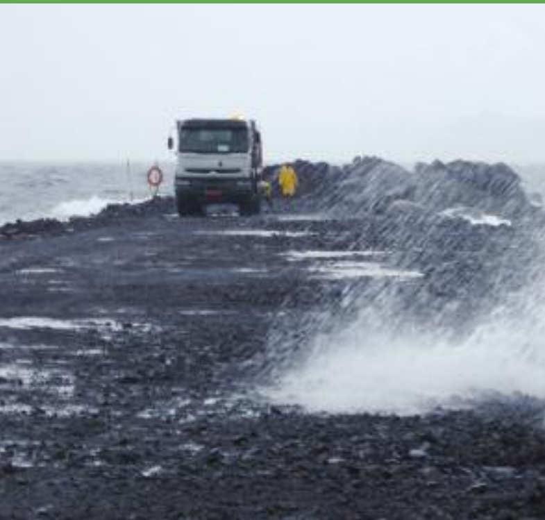
Breakwater construction during rough weather
