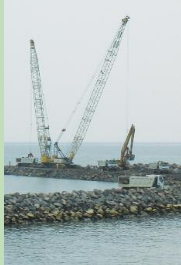
Construction of the breakwater in progress
