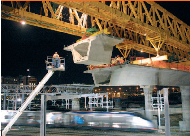
Segment installation above the railway tracks
