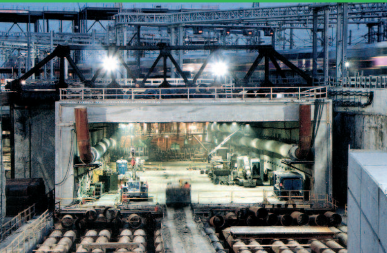
Jack box for I-90 under railway tracks
