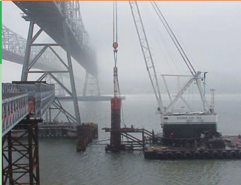
Piling of a 3-metre diameter pile
