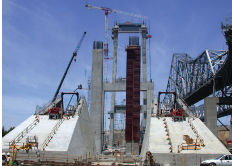
View from the north on completed south anchor
