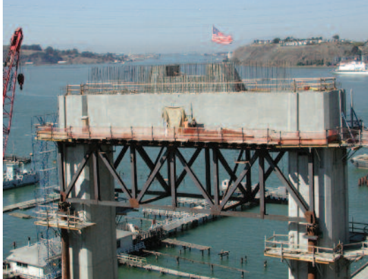
Pier with completed 4-metre-high strut and shear key
