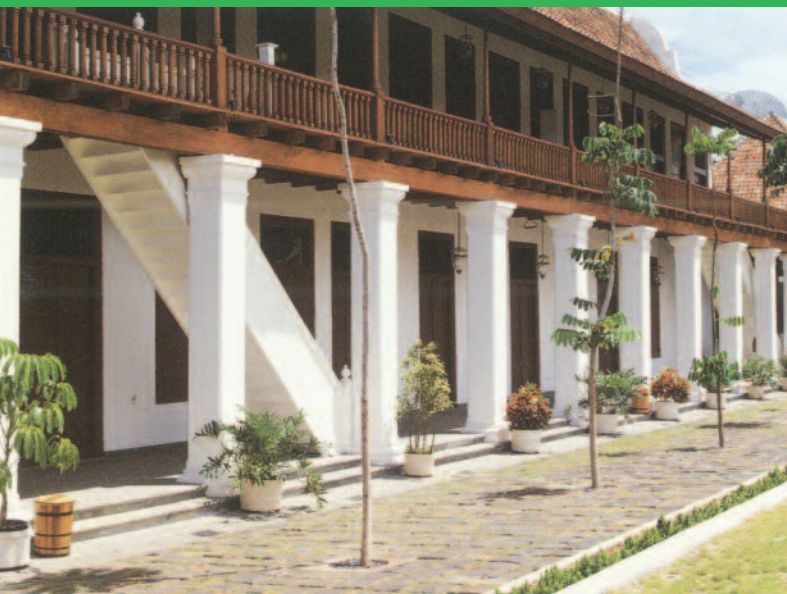
View on Wing building passageway and balustrade of the first floor, both restored in old style
