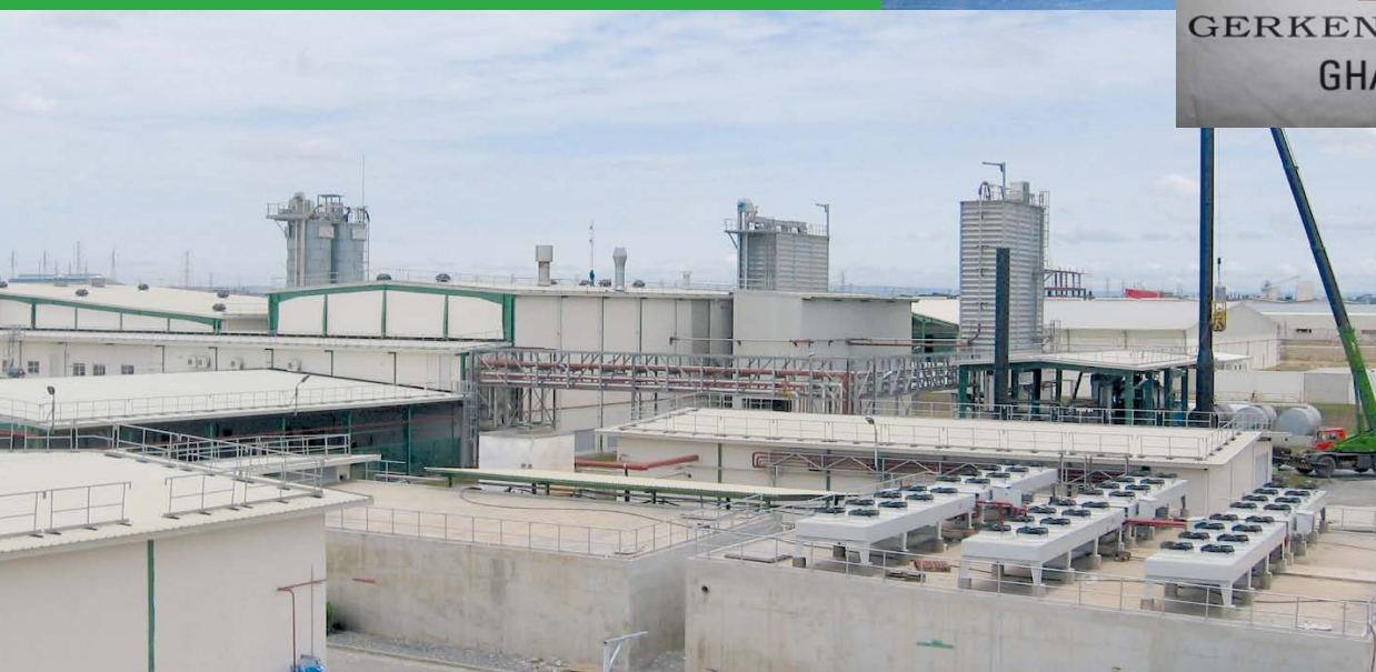
Auxiliary buildings: Sprinkler house, city water tank, compressor house and boiler house
