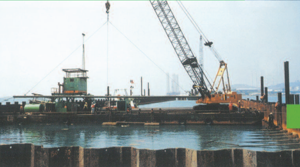
Completed quaywall at inner side of breakwater
