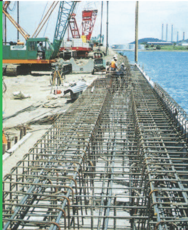
Installation rebar at combi wall
