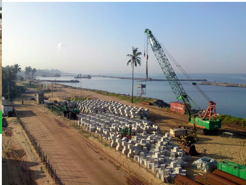
Over 6,000 Xblocs were used for the breakwaters
