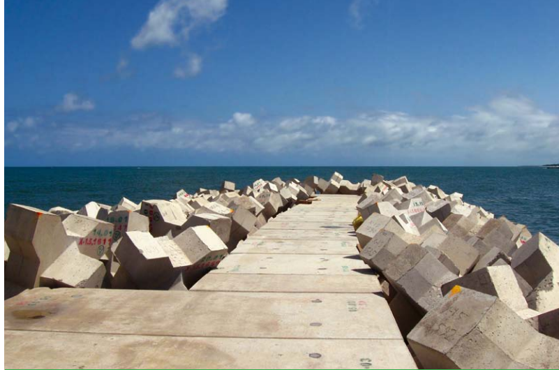
Finished breakwater head
