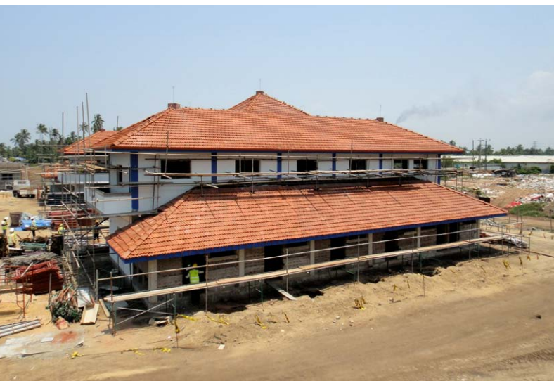
Construction of the main office harbour building
