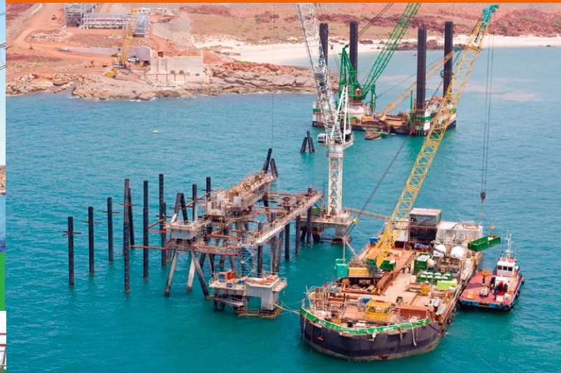
Equipment spread for the platform construction
