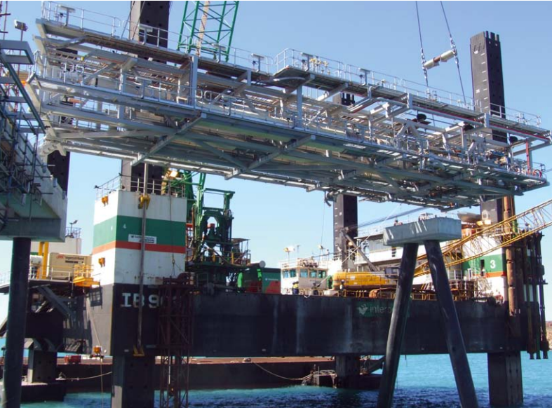
Installation of the first approach trestle
