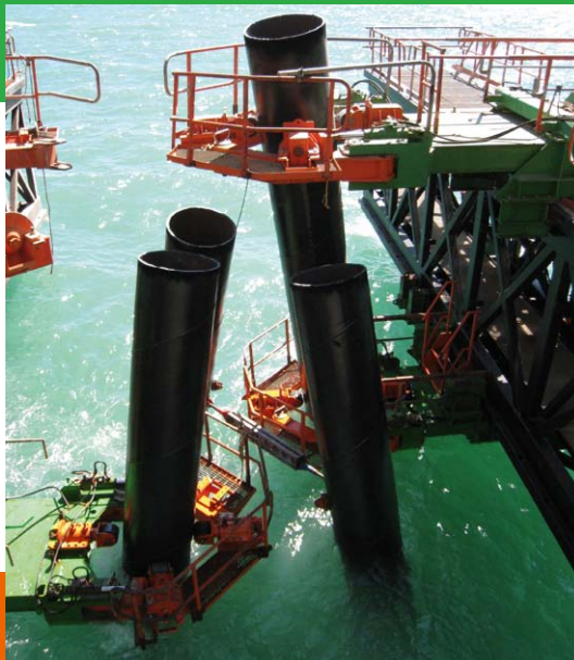
Versatile piling templates on the IB-909
