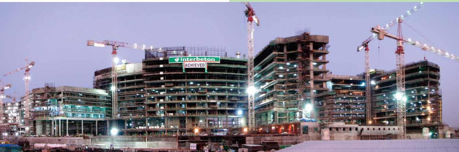
The hotels under construction in November 2008
