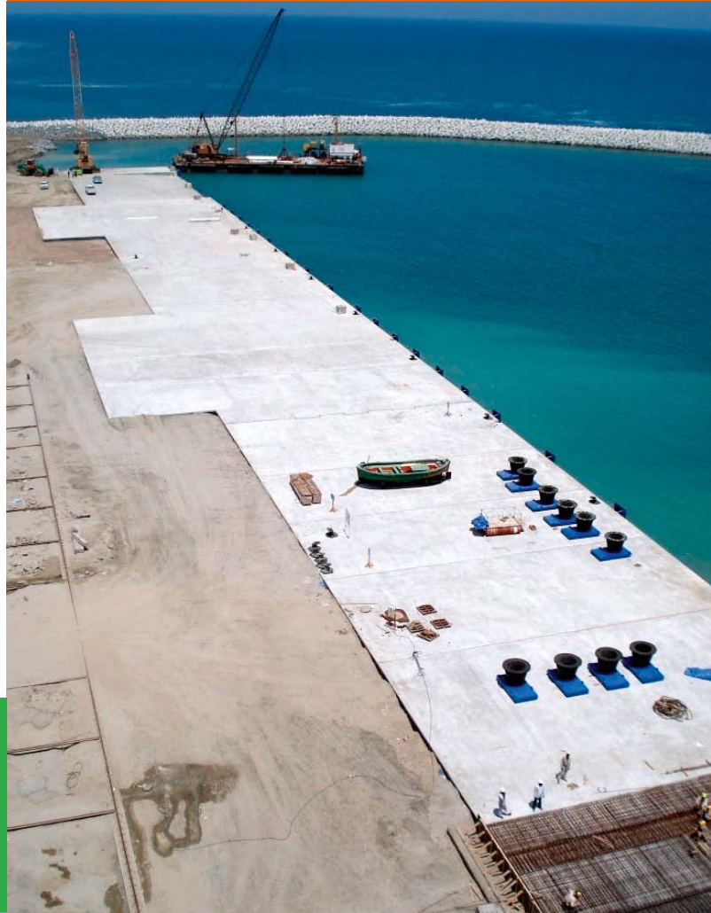
Finishing of the load out platform capable for loads up to 50 ton per m 2
