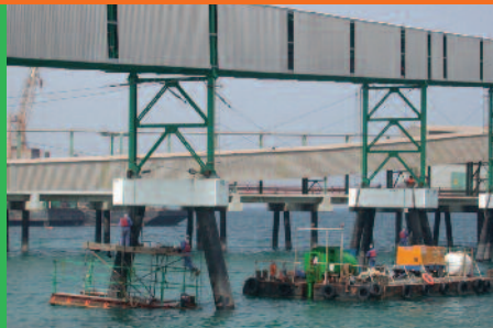
Intermediate conveyor trestle
