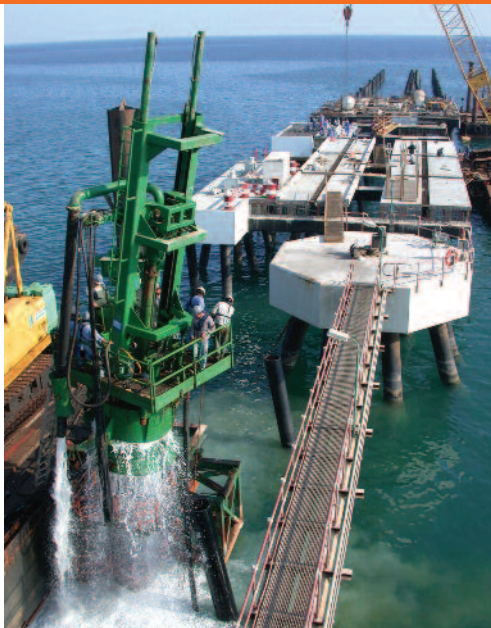
Pile drilling at jetty approach
