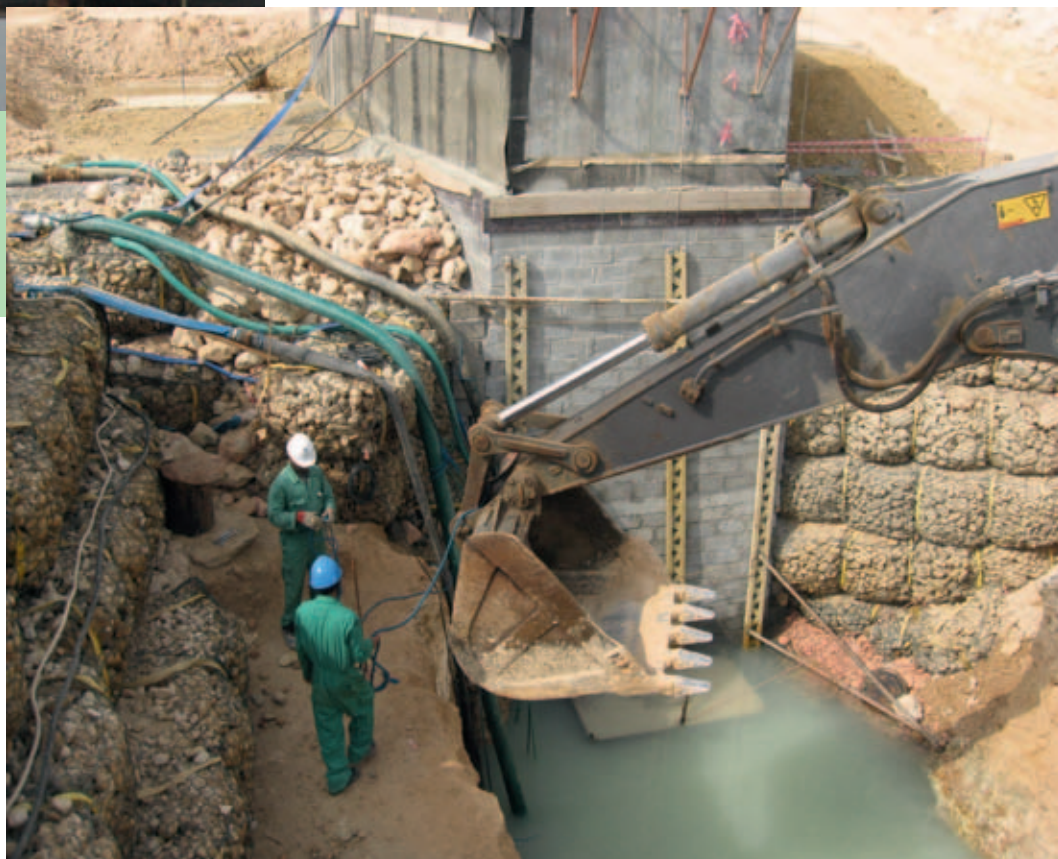
Seawater intake under construction
