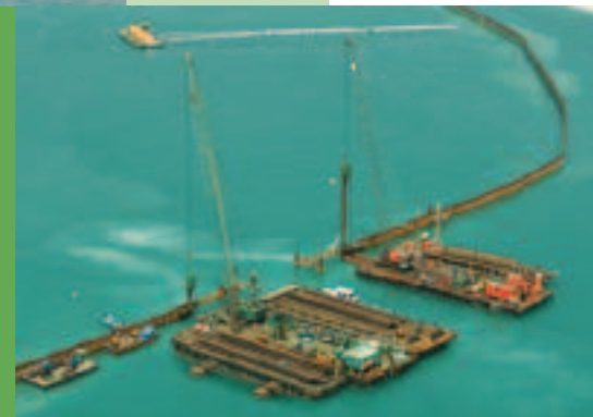
Marine piling in progress
