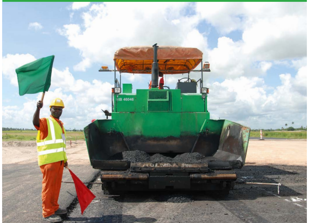
Construction of new taxiways
