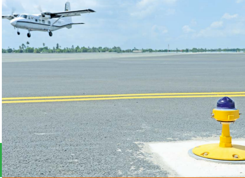
Further upgrading of air ground lighting
