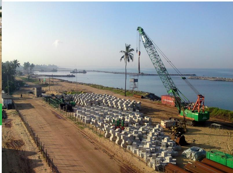
Over 6,000 Xblocs were used for the breakwaters
