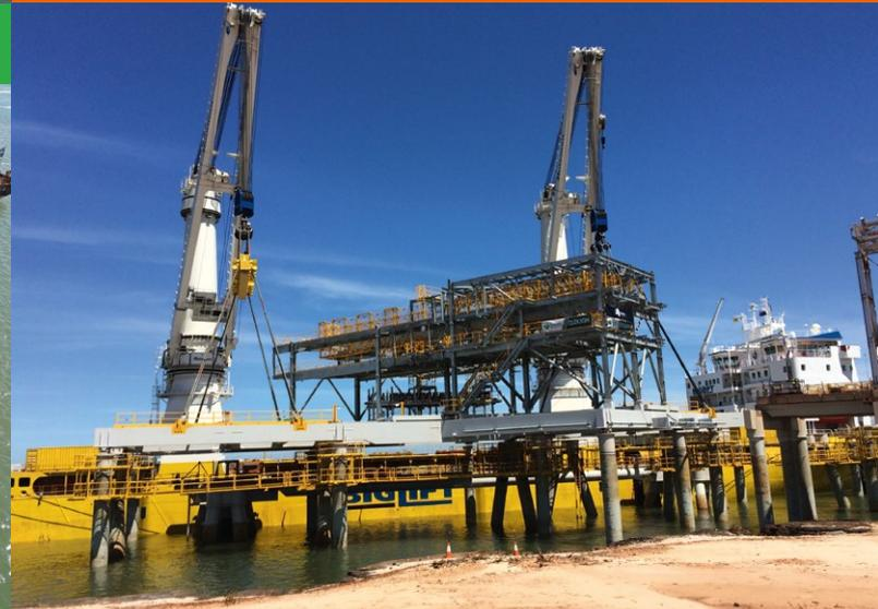
1,500 tonnes in one lift: deck module with pre-installed transfer station
