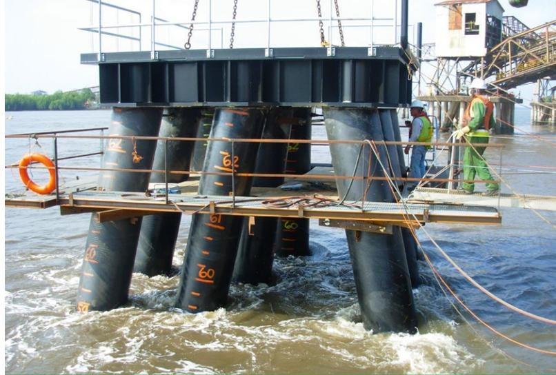
Platform mooring dolphin west placed into position on the piles
