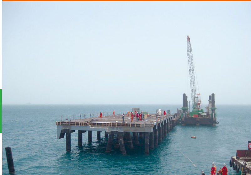
Overview jetty platform under construction
