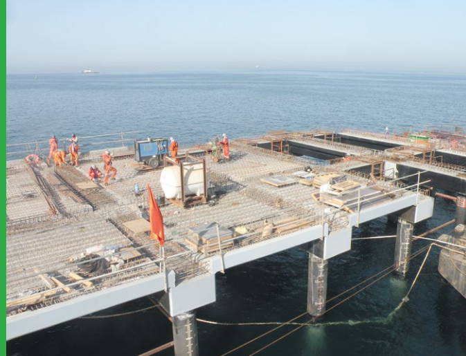
Build-up of jetty deck with precast concrete
