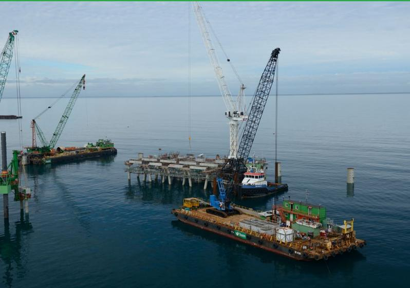
The in-house developed cantilever bridge: building the jetty while standing on the jetty.
