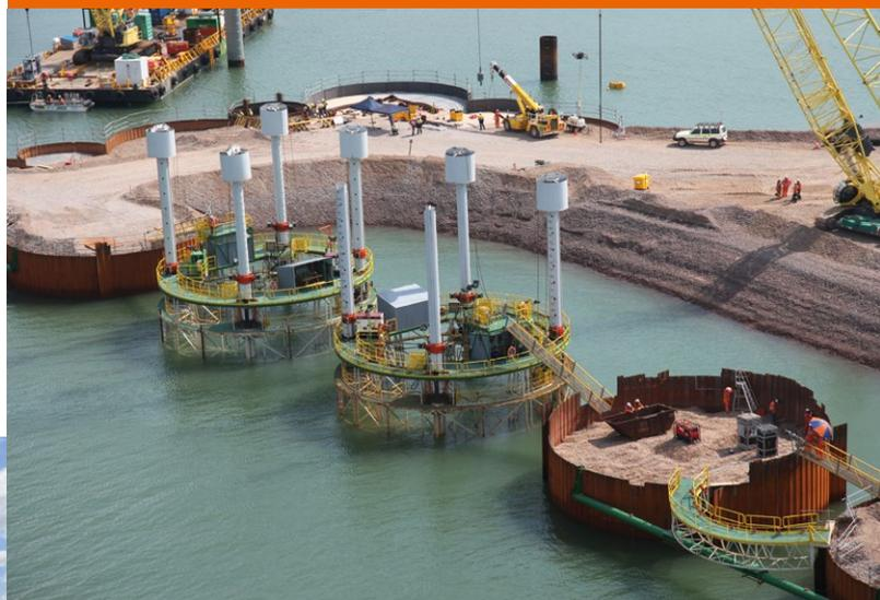
The cell template lowers its four spud legs to the sea bottom and will climb hydraulically free from the barge deck. The sheet piles are pitched around the cell template, held into position and then driven into the seabed. During the placing of the sheet piles, the template and spuds provide stability and rigidity.
