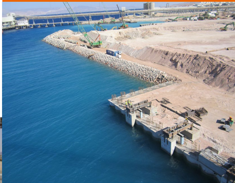
Capping beam construction
