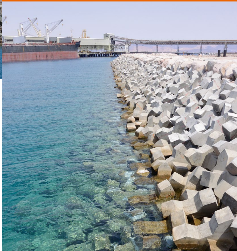
Main revetment – Xbloc primary layer
