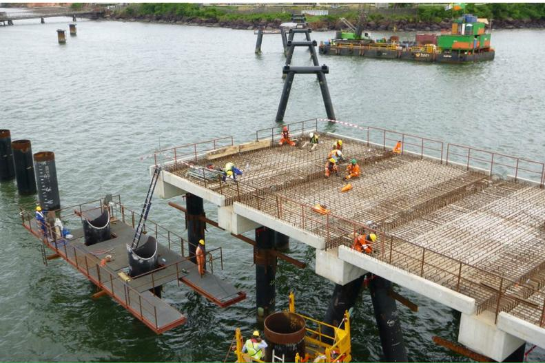
Placing of steel plates on the loading platform
