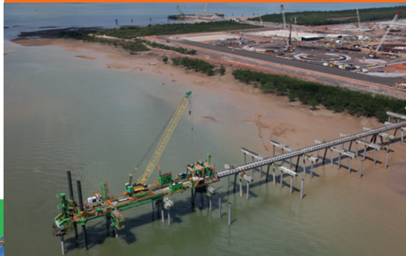
Construction of the jetty
