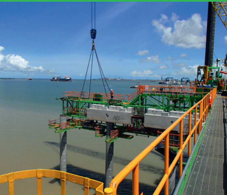
Extended side template of the cantilever bridge
