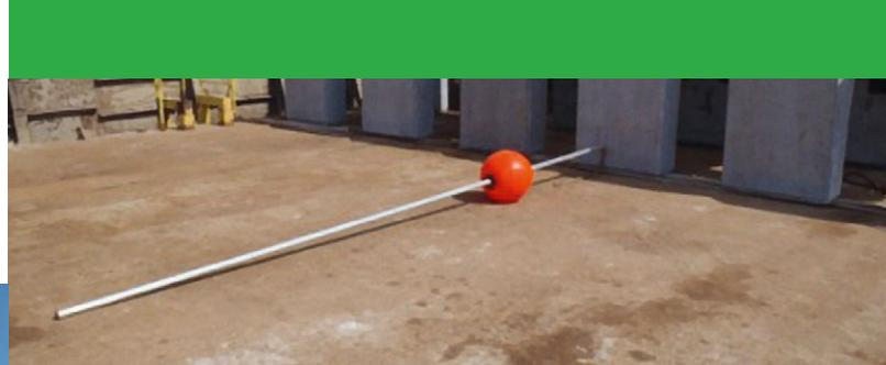
Pencil buoys were attached to the Southern Outfall diffusers. They proved useful for the barge crew to identify the positions of the diffusers during placing of the rock.
